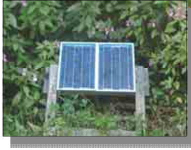
The PV Array powers the garden watering system above
