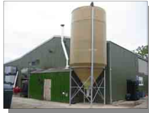
The Pellet Store and Boiler Room at Bethesda Milk's Dairy
